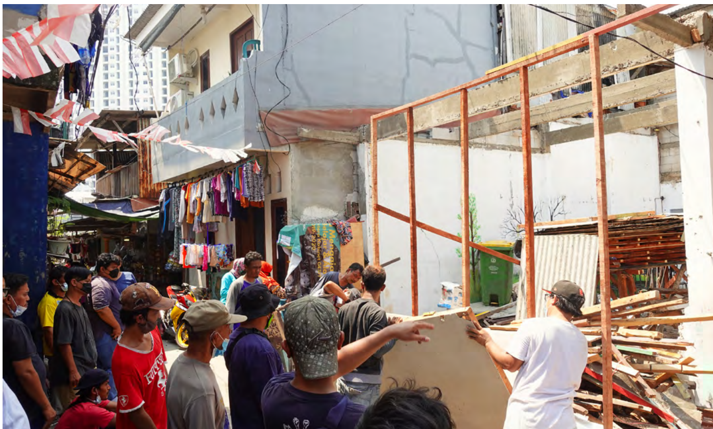
Photography by Urban Poor Network of Jakarta, and Urban Poor Consortium
